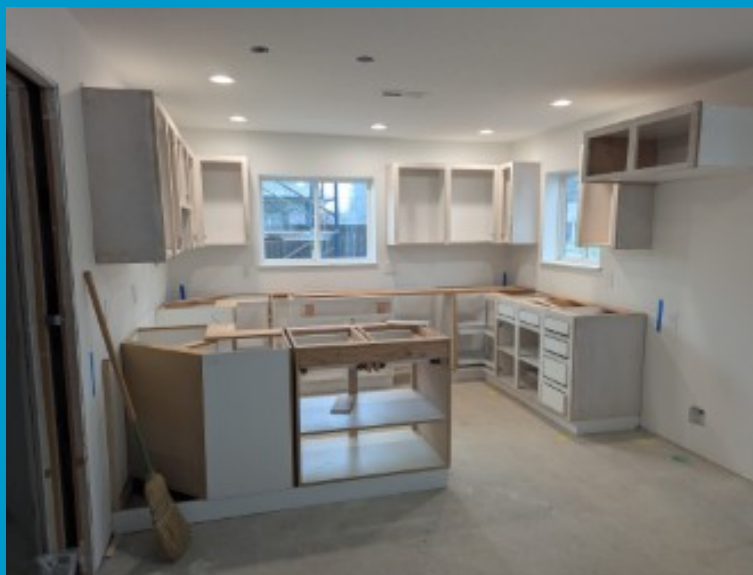
Photo: Cabinets are installed in the 719 Home!
